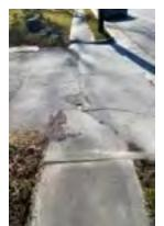
The photo to the left shows a driveway apron/crosswalk that should be improved. It is too broken and uneven. Because we do not provide concrete construction services, this is not work that we can provide. It will require a general contractor.
