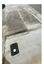
The photo to the left shows an area of sidewalk that should be replaced with new concrete. The surface is spalled, and it is too uneven for a repair. Because we do not provide concrete construction services, this is not work that we can provide. It will require a general contractor.
