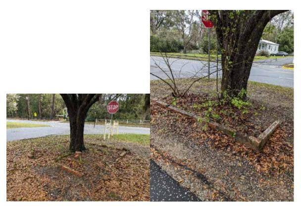
The brick boxes shown above are in a state of disrepair and should be removed. Plants in the planters should be removed as well, leaving the trees to match the rest of the trail. All bricks removed should be preserved to repair the existing planters by Guyton Elementary.
