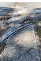
The photo to the left shows where an ADA ramp is needed; however, in the even that the city is unable to construct a ramp, we will cut the curb where it is higher than sidewalk to create a flush joint stepping off the sidewalk. This is a repair that would be included in this repair offer.
